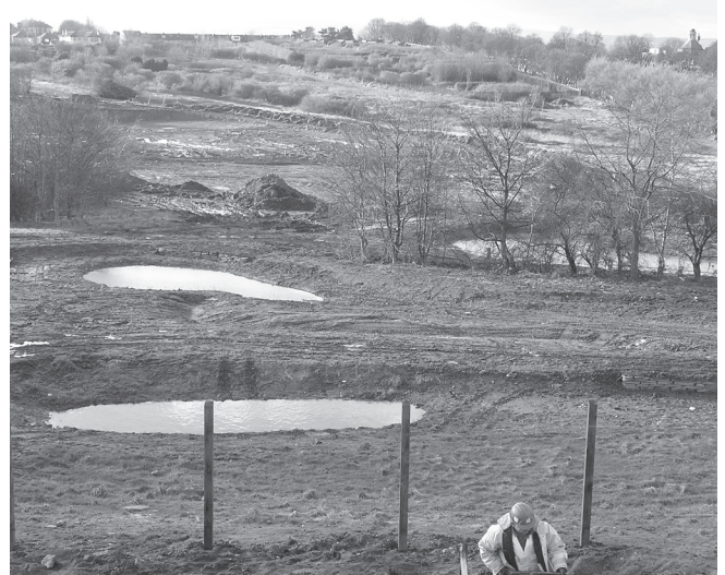
Constructing SUDS in the new Park
