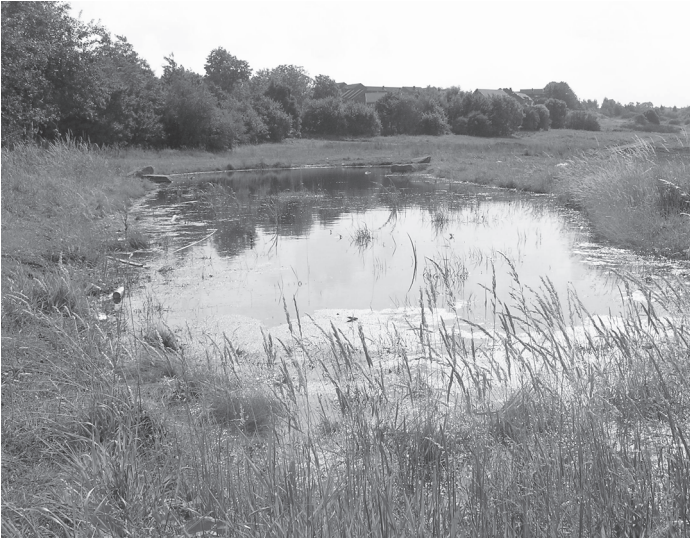
Finished basin in Manor Park
