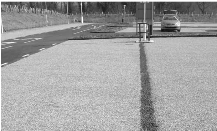
The lorry park site at Farnborough airfield
