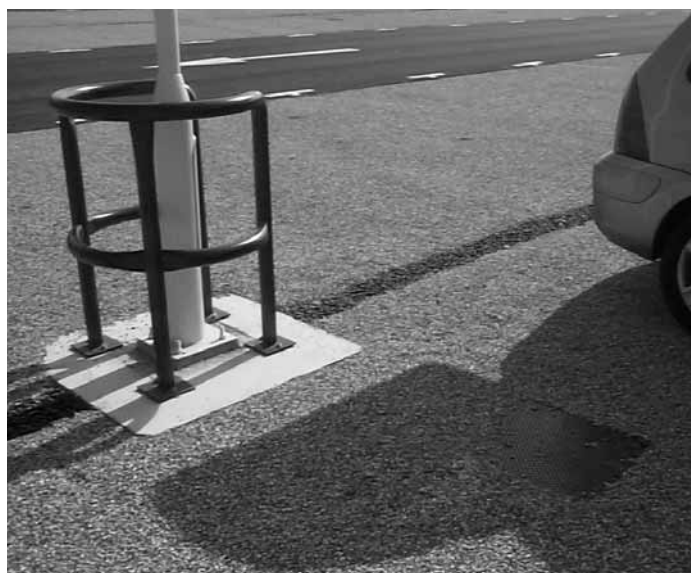
Use of gravel in a porous pavement
