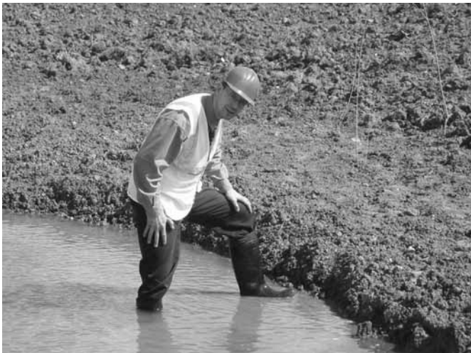
David Singleton checking the marginal shelf on detention basin at Monyhull.
