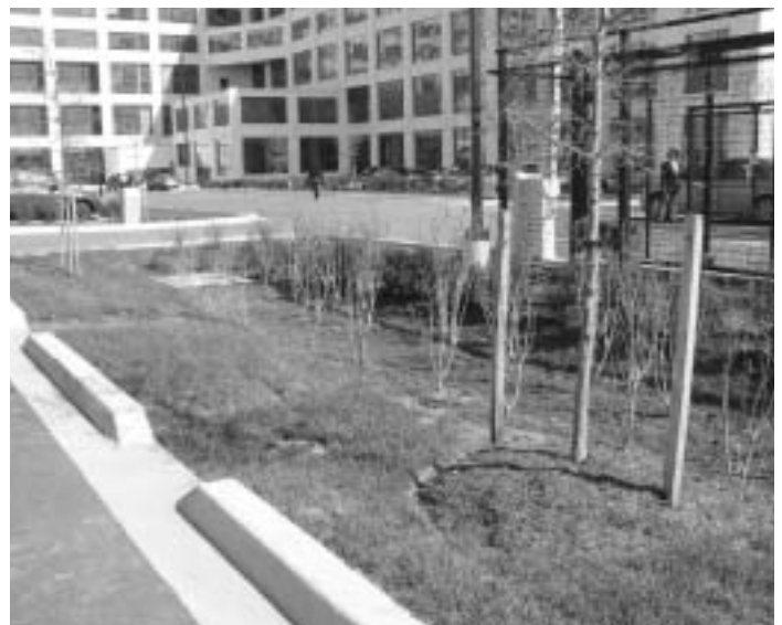
Bioretention areas. Courtesy of SDA
