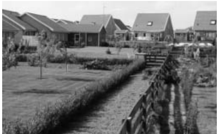
Infiltration trench in Malmö, Sweden. Courtesy of C J Pratt.
