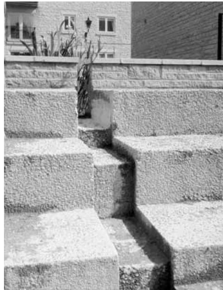
Blashfield Place: Slot well and outfall to discharge to River Welland. Photo: Bob Bray, Robert Bray Associates.
