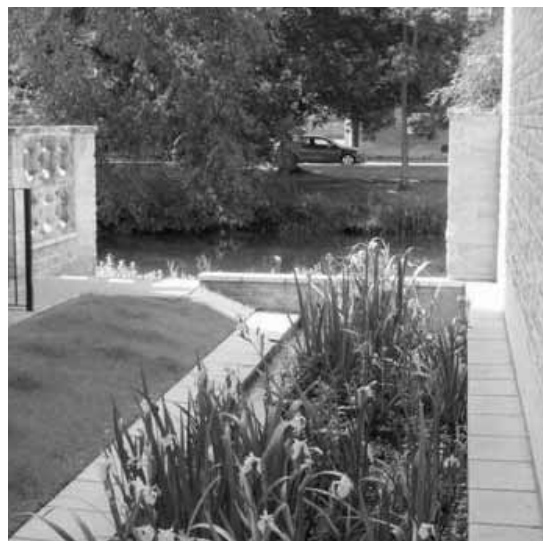
Blashfield Place: A canal part of the conveyance system at Stamford. Photo: Bob Bray, Robert Bray Associates.
