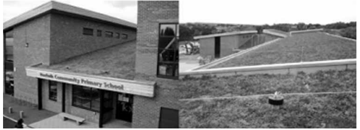
Roof (Courtesy (left) C Basilio (right) Sheffield City Council)
