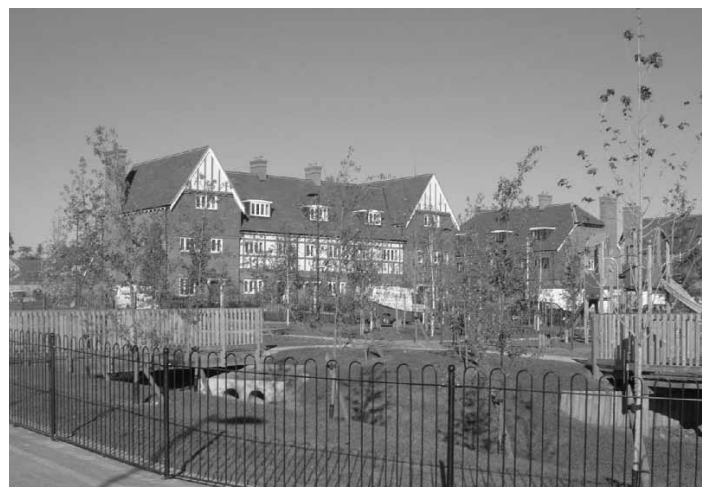
A swale located within the Upton Housing development
