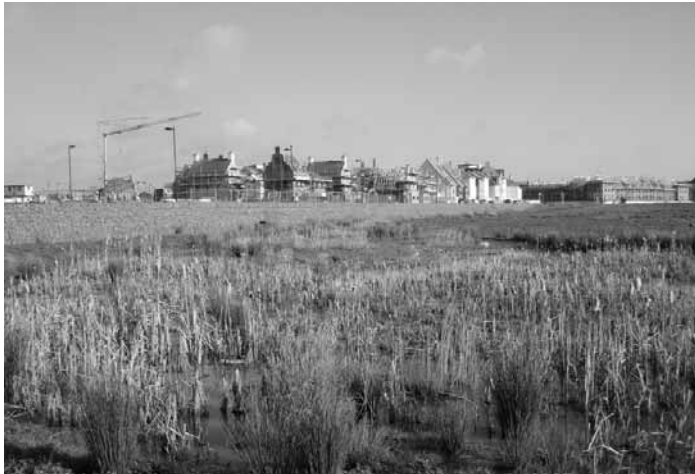
Part of the pond retention systems within the Country Park at Upton.
