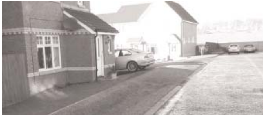
Roadside Swales at West Grange Development, Dundee. Courtesy of SISTech
