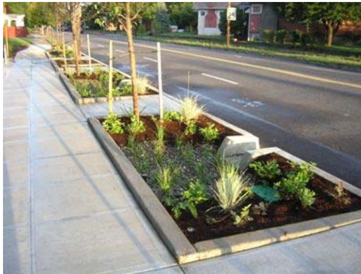
Figure 2: Surface water planter box in Portland, Oregon.
