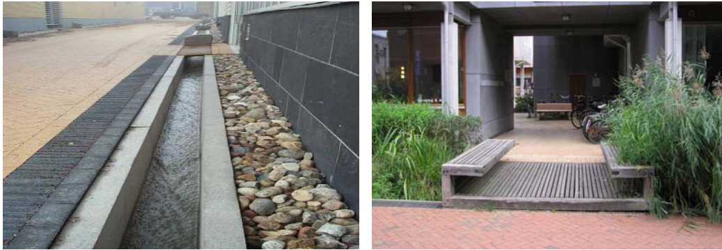
Figure 5 – examples of hard (left) and soft (right) drainage features in dense urban environments in Malmo.
