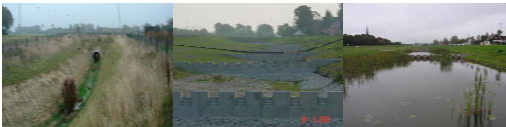
Figure 4 – Example of improvement to stormwater drainage from an industrial area. Images show the original structure (left), the improved structure (centre) and the improved structure providing retention following a storm event (right).
