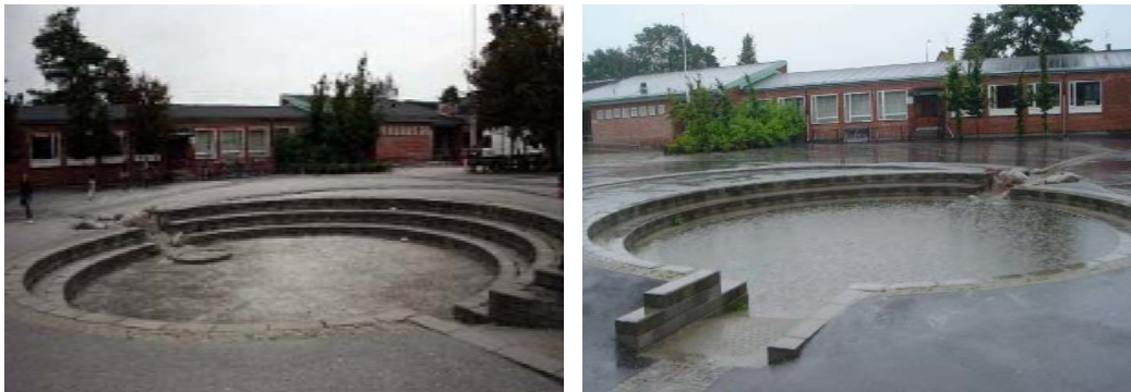
Figure 3 – a school playground amphitheatre also functioning as a storage structure for 1 in 10 year storm events.
