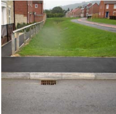
Figure 3 Poor detailing of a swale
