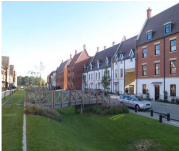
Figure 1: A swale at Upton, Northampton
