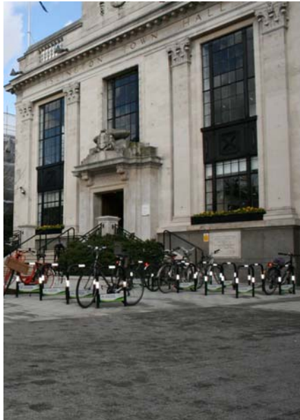
Figure 7 Permeable paving, Islington Town Hall
