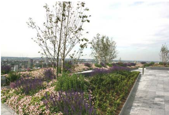
Figure 6 Green roof and photovoltaics (Ropemaker)
