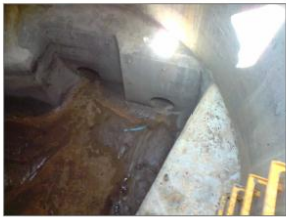
SURFACE WATER MANHOLE – S70 DEPTH TO INVERT APPROX 2.95 DESIGNED 1 X 240mm ORIFICE AS BUILT = 2 X 240mm ORIFICES
