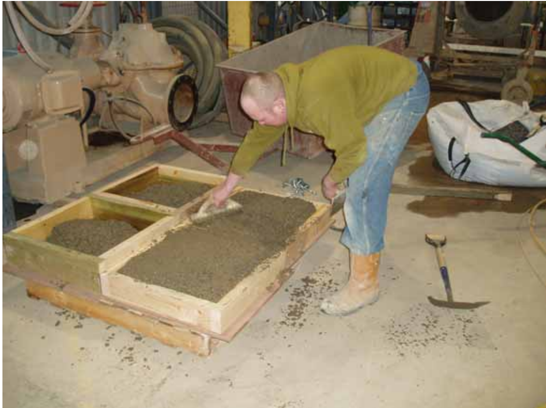
Photo 9.1 Casting floor slabs
