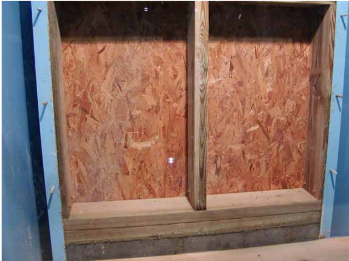
Photo 7.15 Wall TF1 being built showing OSB - view from inside
