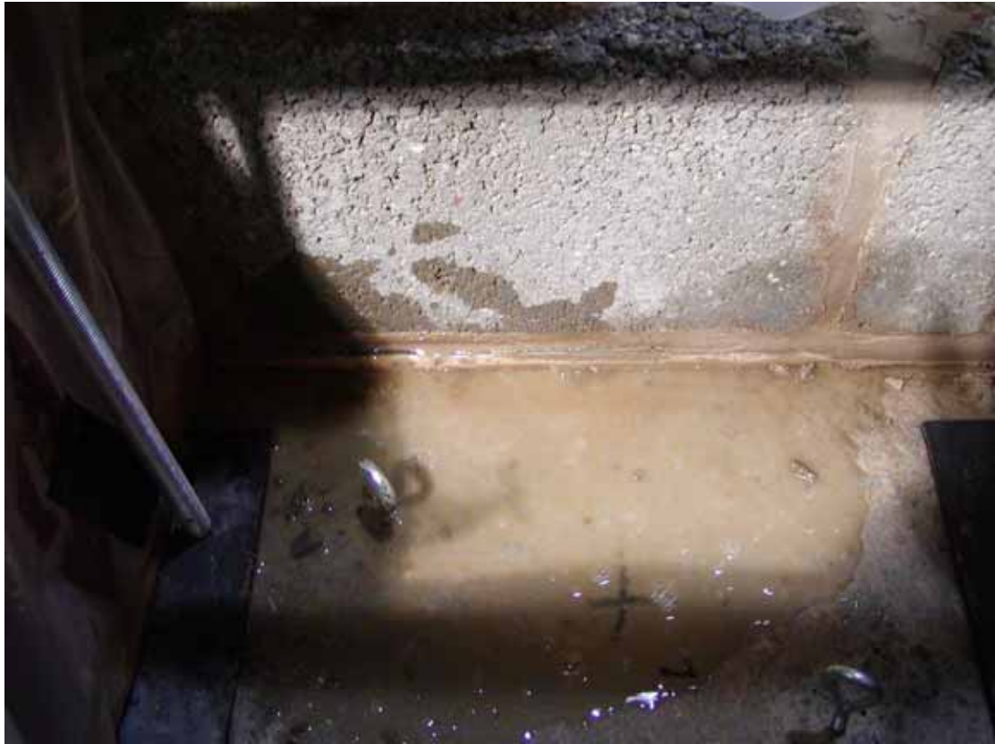
Photo 9.7 Floor Arrangement 6; leakage through wall- floor junction
