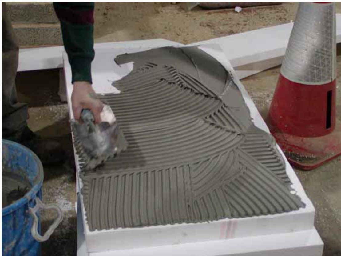
Photo 10.7 Wall S4.2 - Wall with external insulation; applying the insulation
