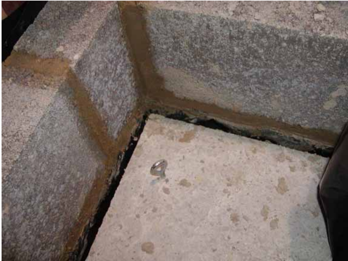
Photo 9.9 Arrangement 8; Wallfloor corner joint
