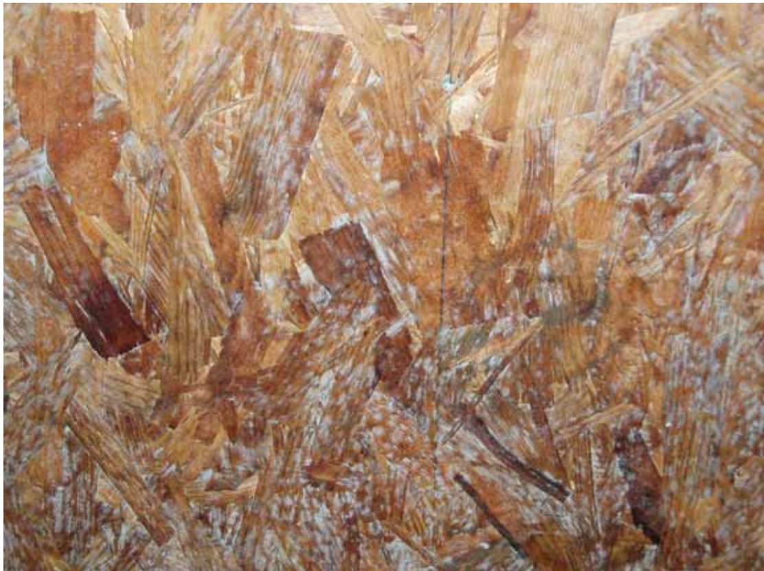
Photo 7.22 Mould growth on timber sheathing
