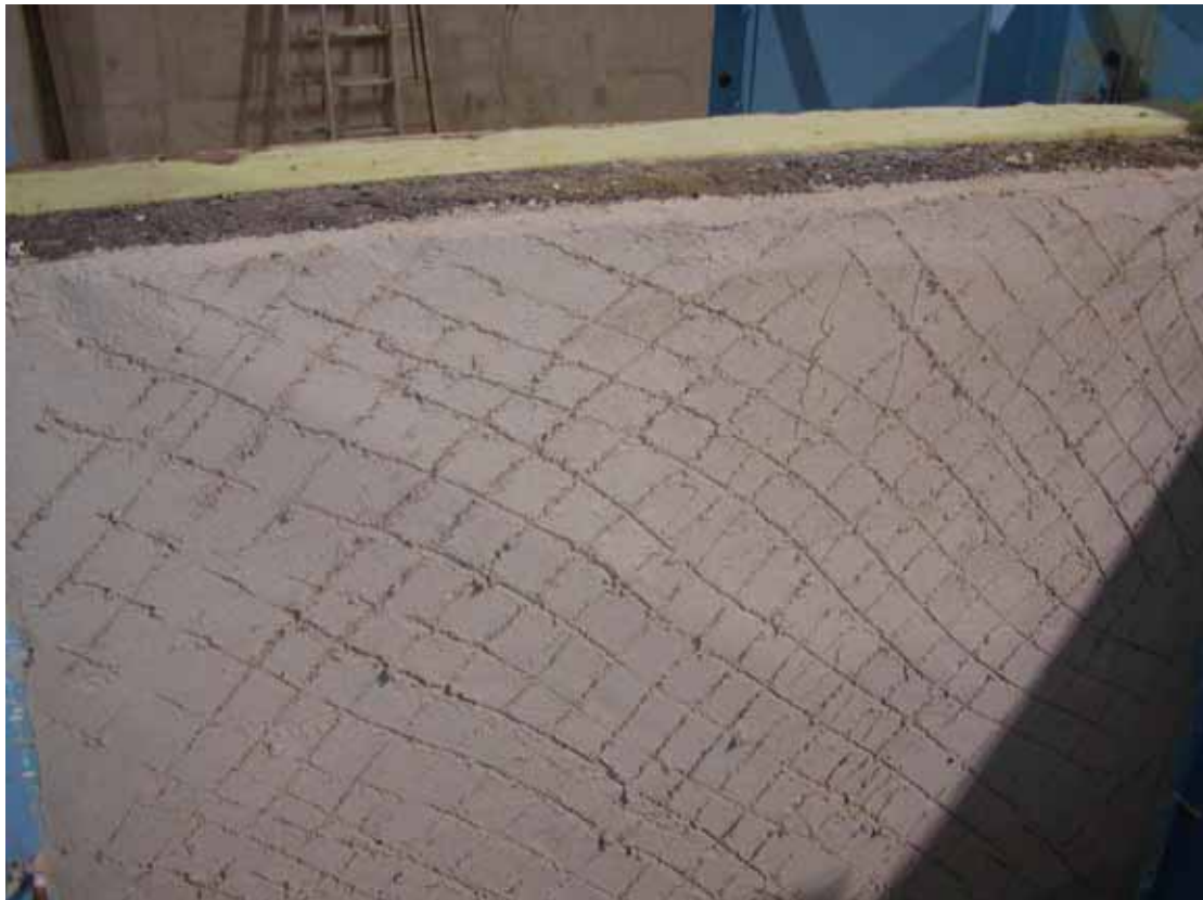
Photo 7.18 Wall ME5; first coat of render
