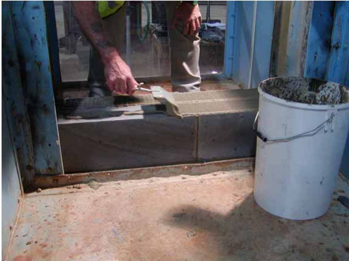
Photo 10.2 Wall S4.1 - Applying mortar on thin joint wall
