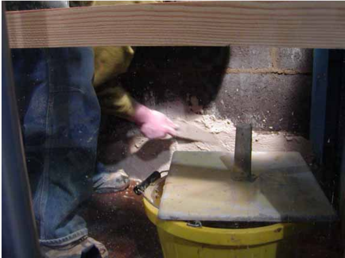
Photo 7.19 Wall MFF3 Applying lime plaster
