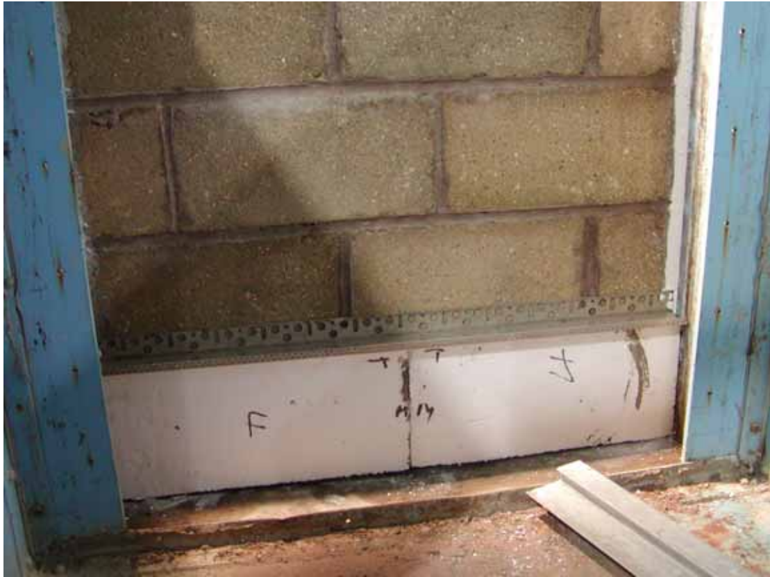
Photo 10.6 Wall S4.2 - Wall with external insulation; insulation placed below DPC level
