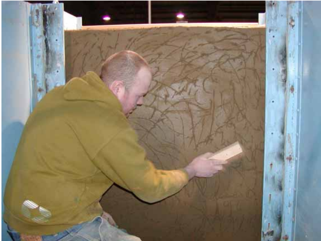
Photo 7.17 Walls TF2 and TF3; applying external render
