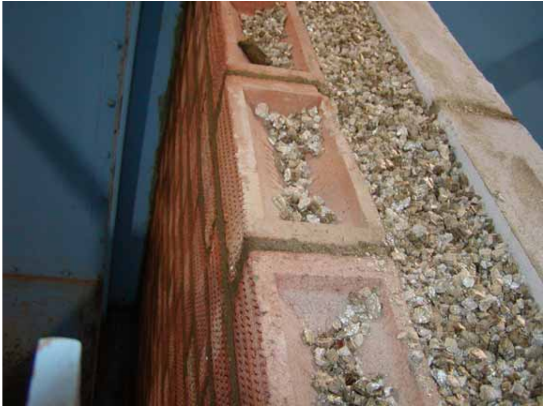
Photo 7.9 Wall MFF2 showing loose insulation in cavity after construction
