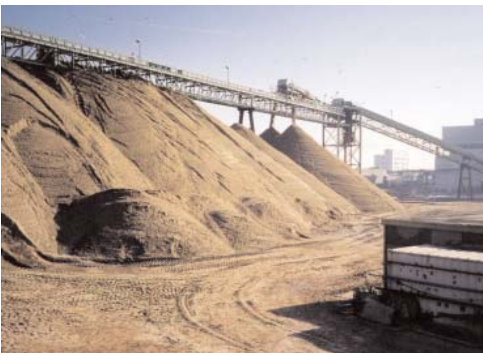
Marine aggregate at Hanson Aggregates Nederland NV, Amsterdam
