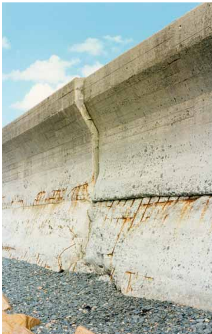
Concrete wall, Jersey (courtesy HR Wallingford)
