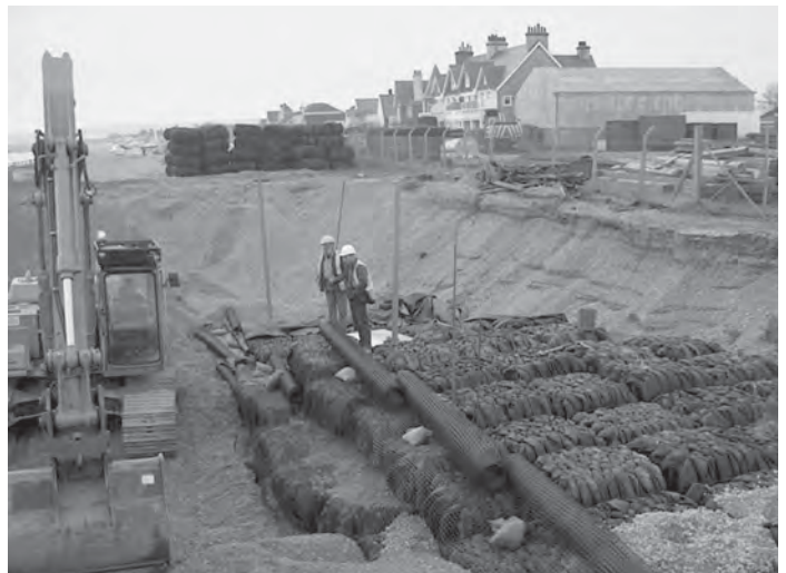
Tyre bales being buried at Pevensey beach (photo: Pevensey Coastal Defence)
