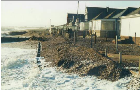
Figure 1: Typical erosion prior to improvement works
