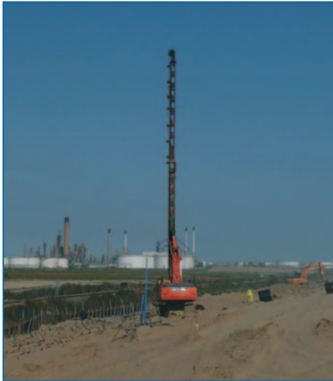
Figure 2 Vibro compaction machine
