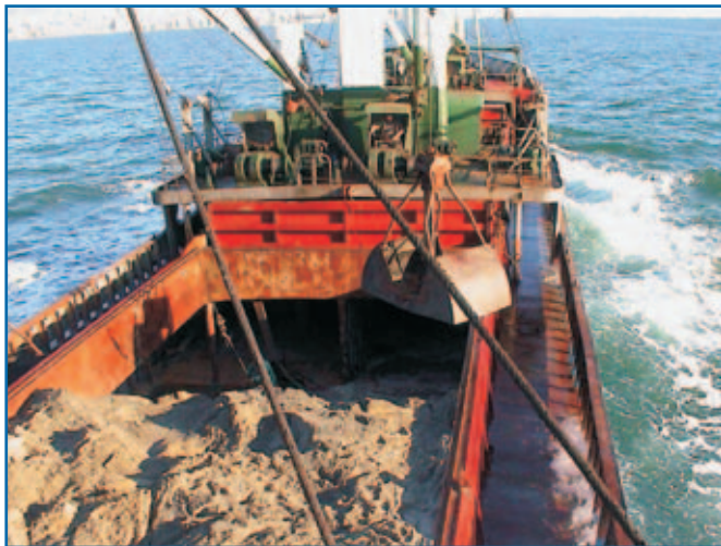
Figure 7 Clam shell dredging
