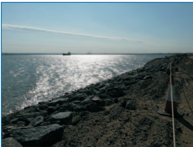
Figure 1 Dredged hydraulic fill
