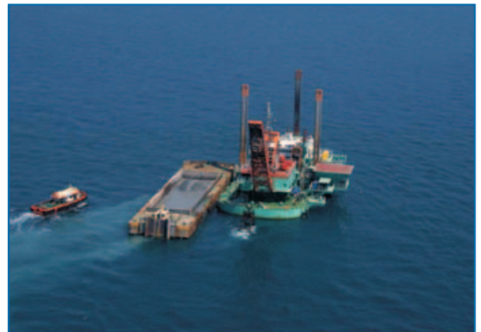
Figure 12 During the dredging
